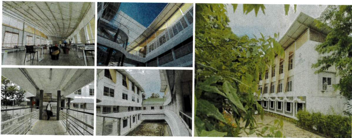
Smart Building Design applied to minimize energy consumption- Cross-Ventilation for classroom, Maximize Daylight: Large windows, skylights, and light shelves bring in natural light via classroom and corridor
